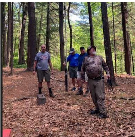
Antenna Crew taking down the R5
